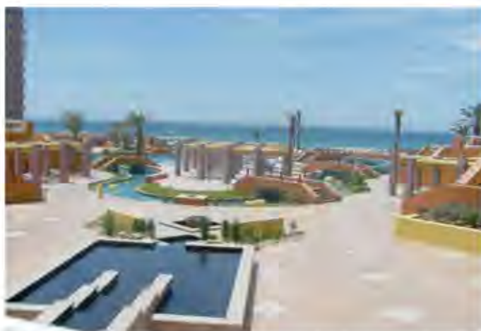
150 Blvd Costero at Rubi Building.
